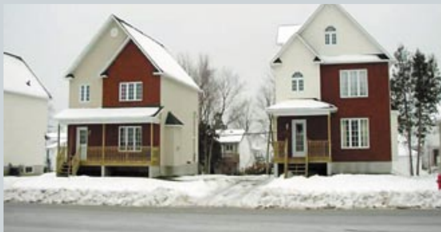
Photos : Construction Chartro
